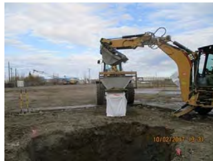
Excavation at Site SS014
